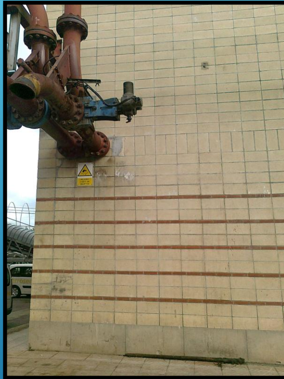
HIGH PRESSURE VALVES – DEGREMONT – VALENCIA'S WATER TREATMENT PLANT – ACTIVATE SLUDGE PLANT -DEGREMONT YEAR 2005
