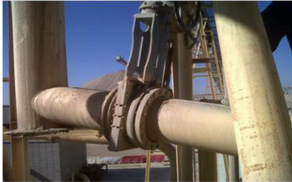
Copper mining, valve DN250, Chile
